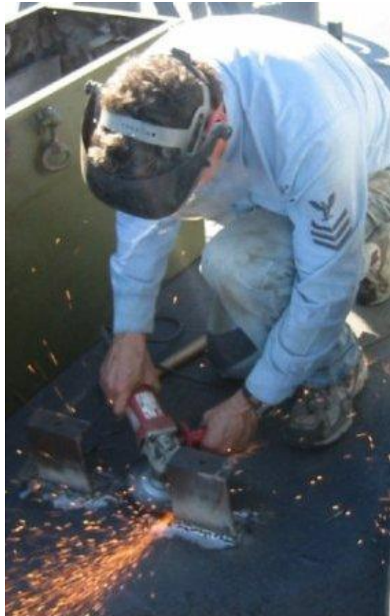
Joe Breyer works on attaching new deck mounts for a refurbished 20mm ammo box.
