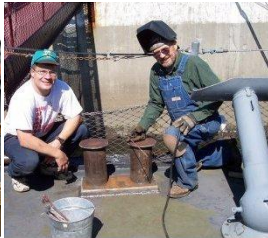
Joe and Tom Schriener welding down the bitts.
