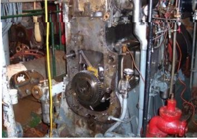
b Gus's beloved emergency diesel in pieces.
