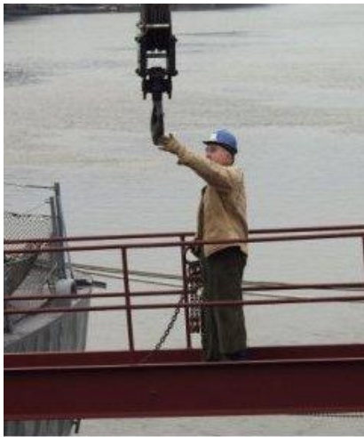
Doug makes the gangway hookup.
