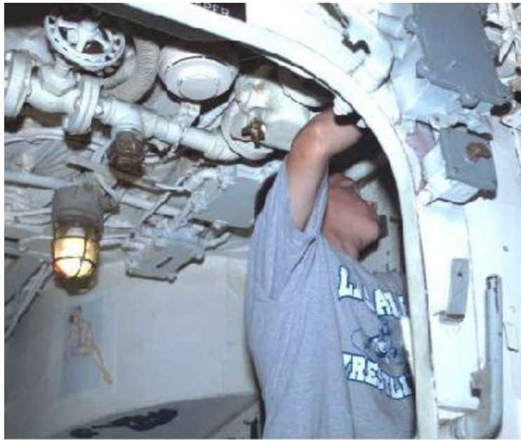
Mike Clark working on alarm wiring.
