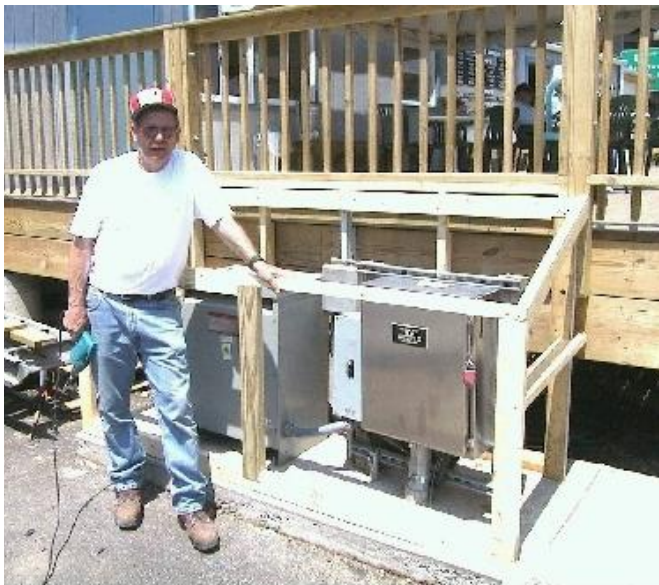
Bob Kibbey working on the power shed.
