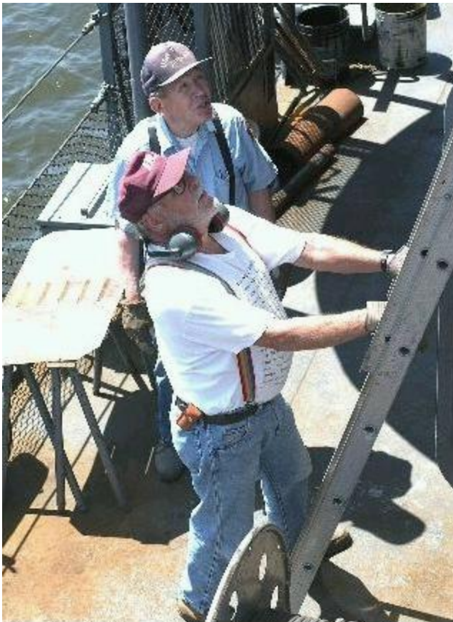
How the hell does he expect me to paint that. Chris Fedden and Ray Lammers rig a ladder to get under a director tub.
