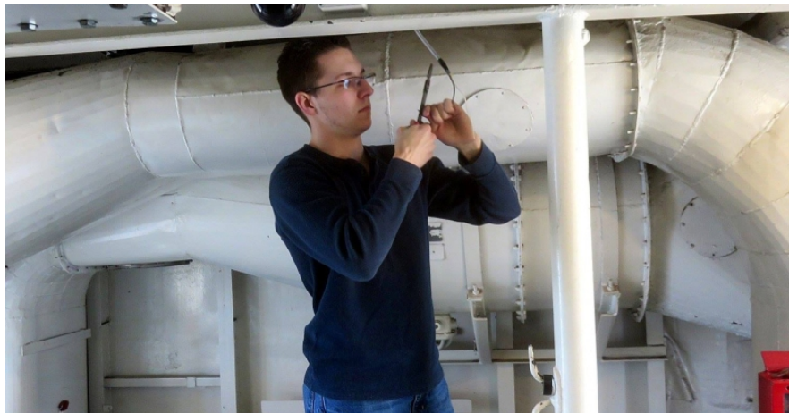
Devon Urbano has been one of our Saturday regulars, assisting Barry Witte with electrical projects.
