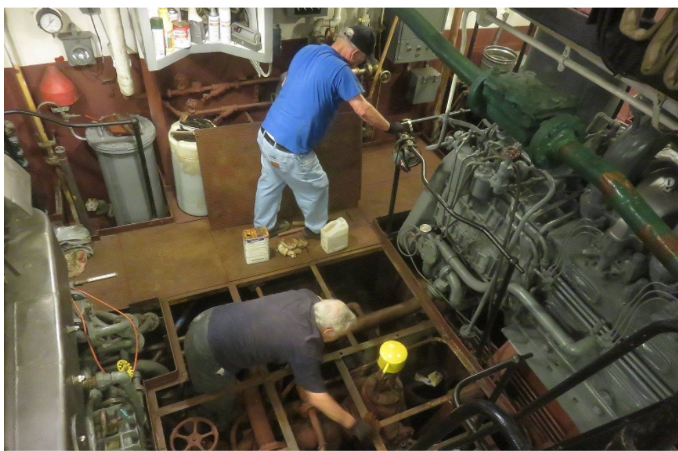
The twins, Karl and Earl Herchenroder, bolting down deckplates.
