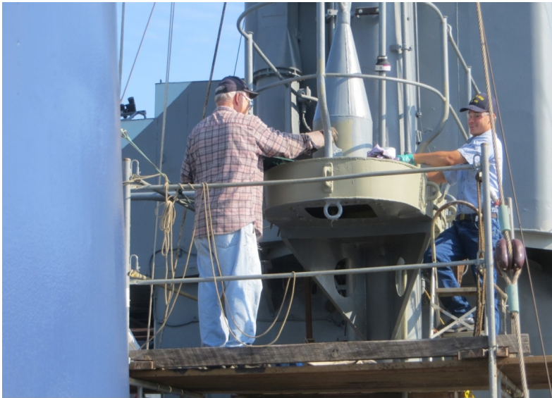
The final coat of paint.
