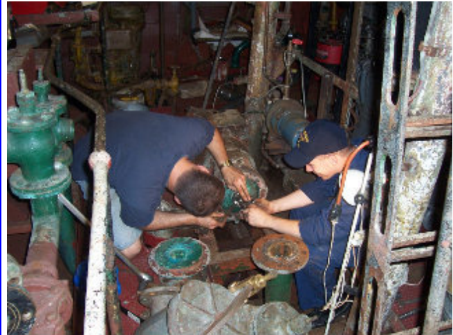
Barry Witte and Mike Fitzgerald overhaul the fire and flushing pump.
