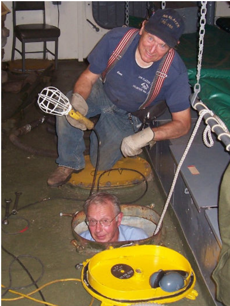
Gene Jackey and Ron Mazure replace a ladder in the starboard fresh water tank.
