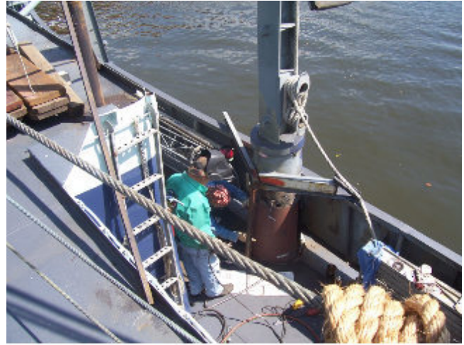
Doug Tanner fitting in the replacement piece.
