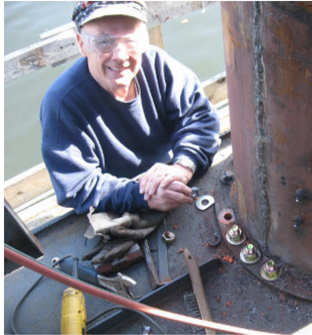
Super Dave Mardon installing new bolts on the davit pedestal.
