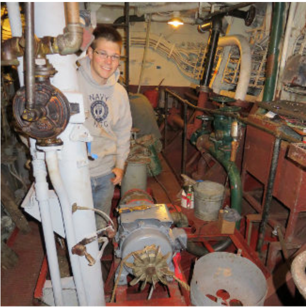
Work continues on the B-3 fire and flushing pump.
