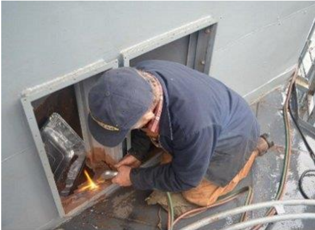
Laird Confer working on the forward exhaust fan room...
