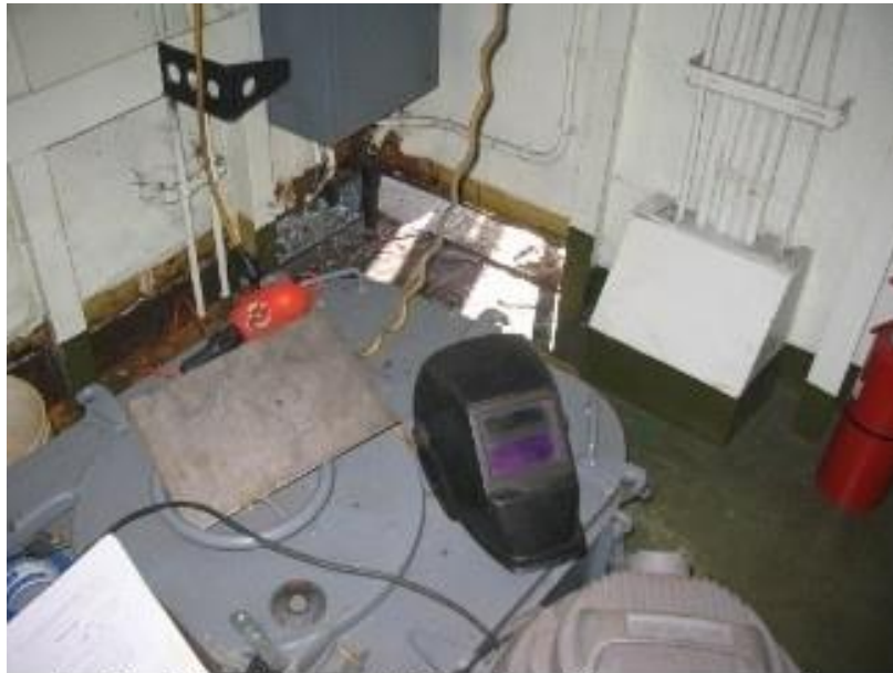
The inside view of the deckhouse steel replacement.
