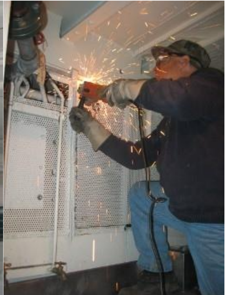
Super Dave starting the scullery restoration.
