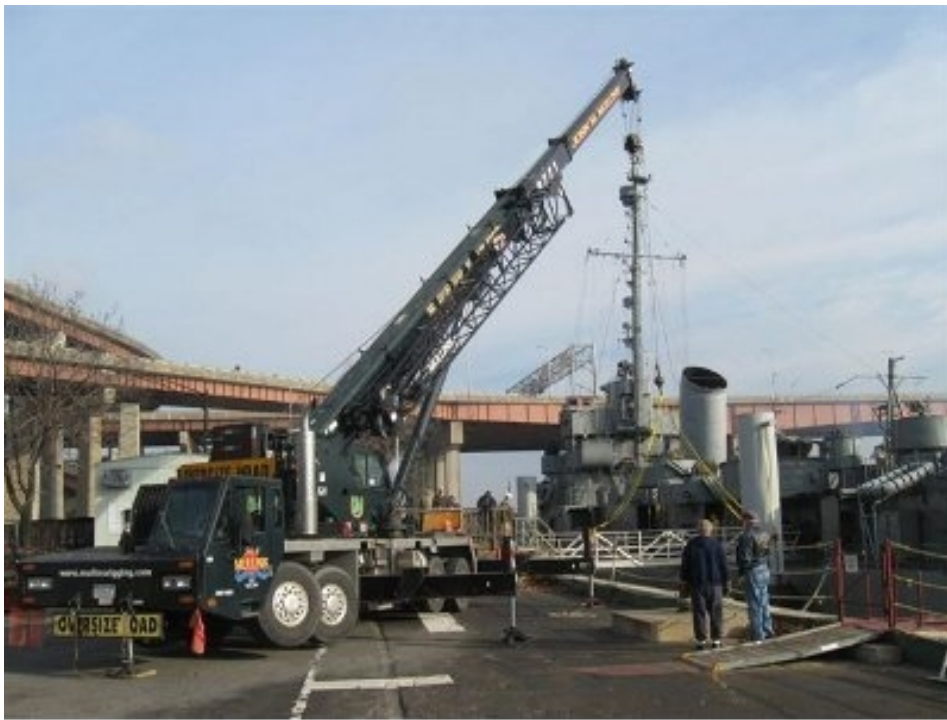
Thanks Marty! Mullin's Crane service to our rescue.
