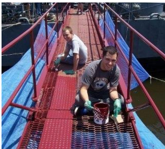
Sailors from the Nuclear Power Training Unit painting the gangway.
