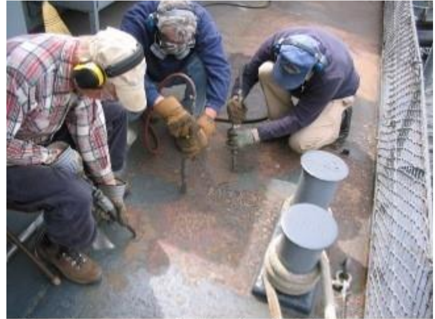
Ron Mazure leads the deck chippers.
