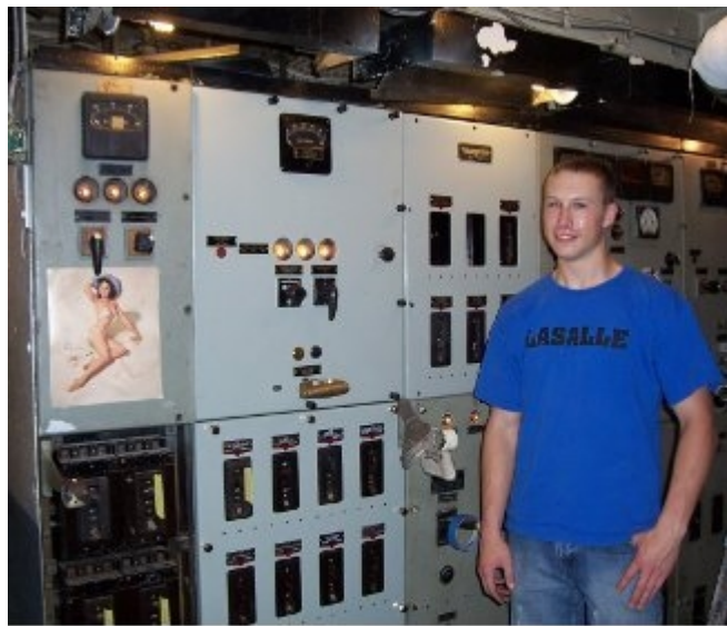
James Conlon shows off the progress restoring the Aft distribution board.
