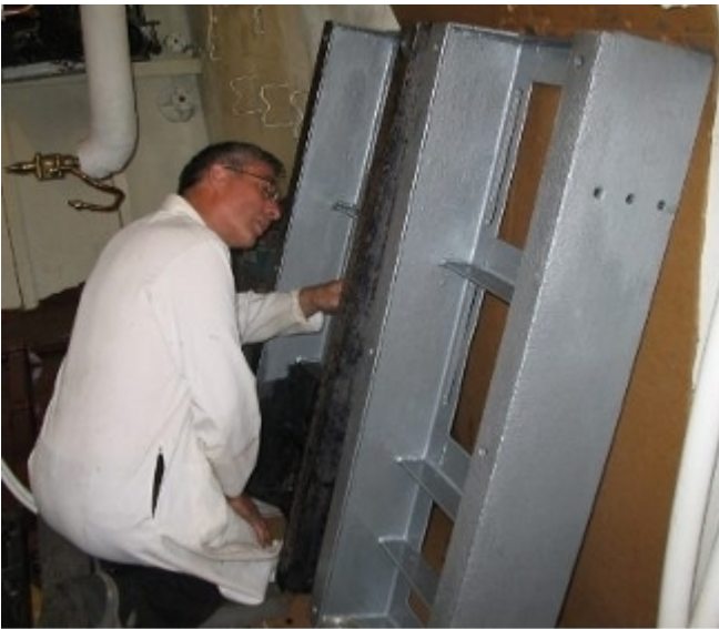
Gary Sheedy repainting the refrigeration compressor bases on the reefer deck.
