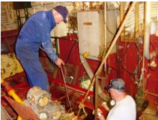
Guy Huse supervising the fire and bilge pump reassembly.
