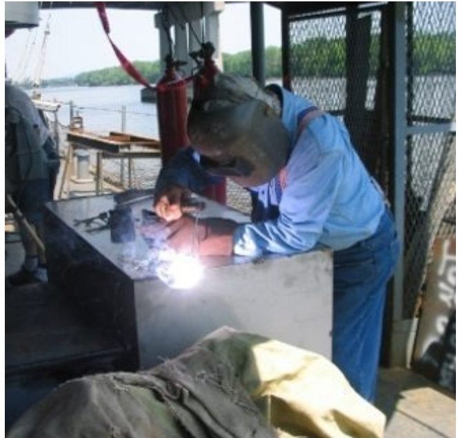
Clark Farnsworth welding on the septic tank for the forward head.
