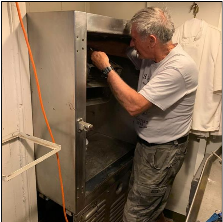
Gary Sheedy mounting a compressor in the wardroom pantry refrigerator.
