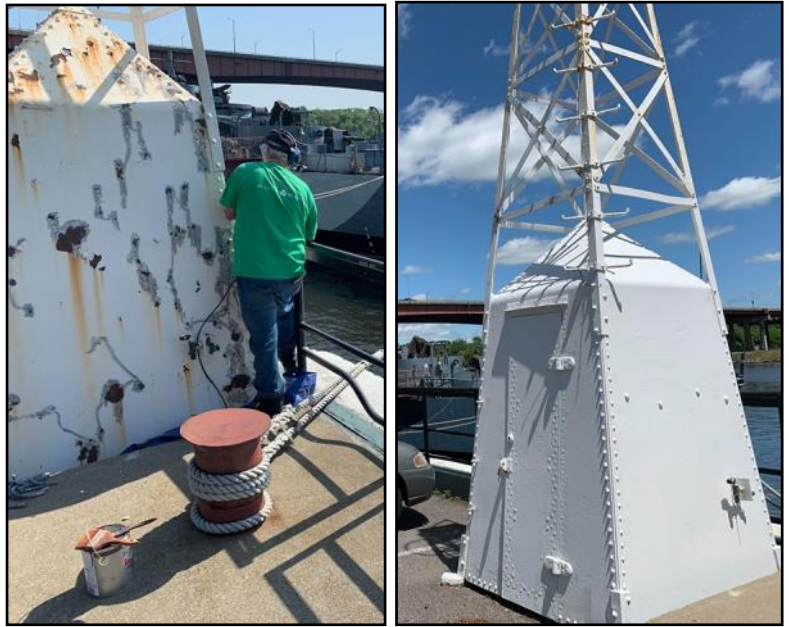
Earl Herchenroder scaled and painted the navigation tower base.
