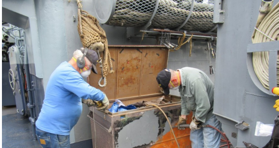
Earl and Chuck scaling the deck gear lockers.
