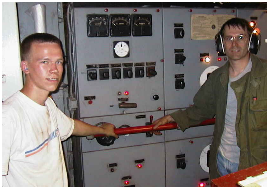
Electricians Mike Clark and Barry Witte.
