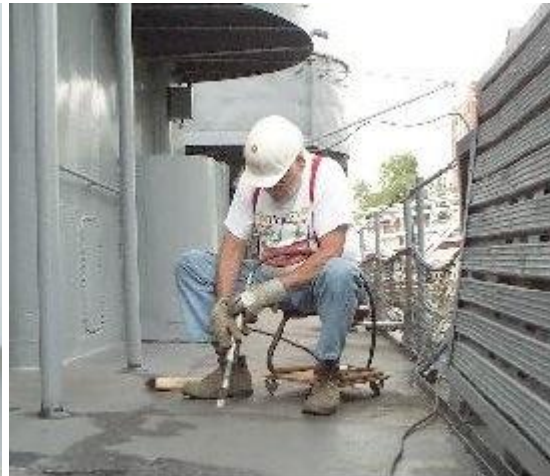
Chris Fedden chipping on the portside main deck.
