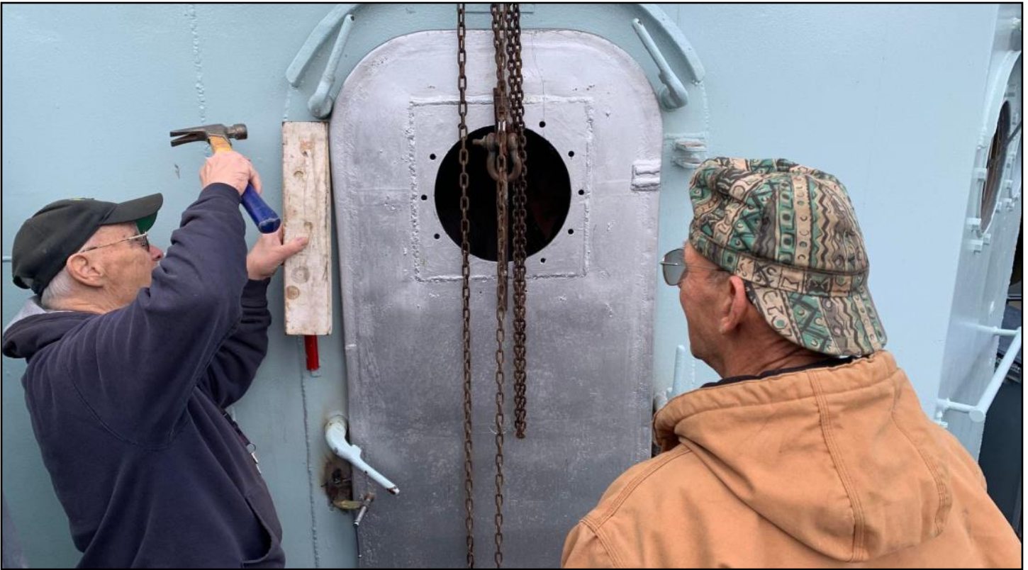
Dave Mardon and Tim Benner are determined to beat the watertight door until it fits.
