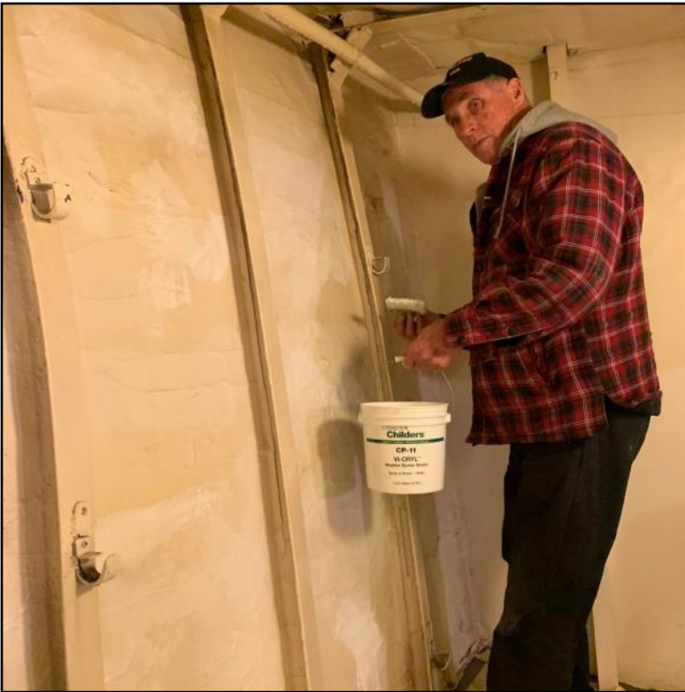
Gary Sheedy repairing insulation in the forward berthing compartment.
