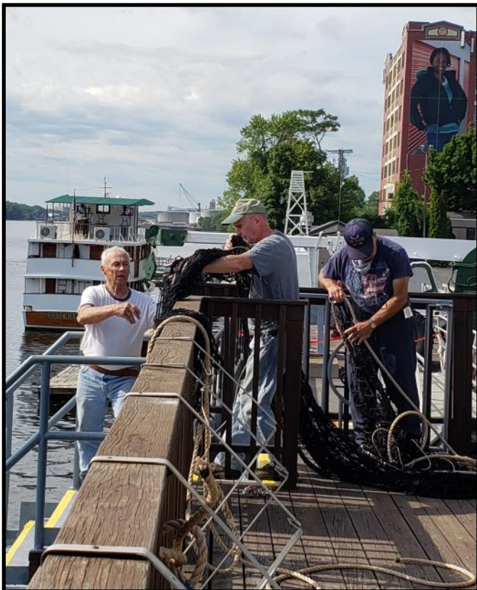
Dave, Chuck, and Doug installing the safety nets.
