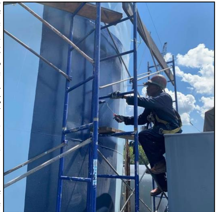
Finishing the painting on the stack.
