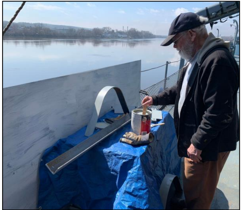
Earl primed metal for the flying bridge repairs.
