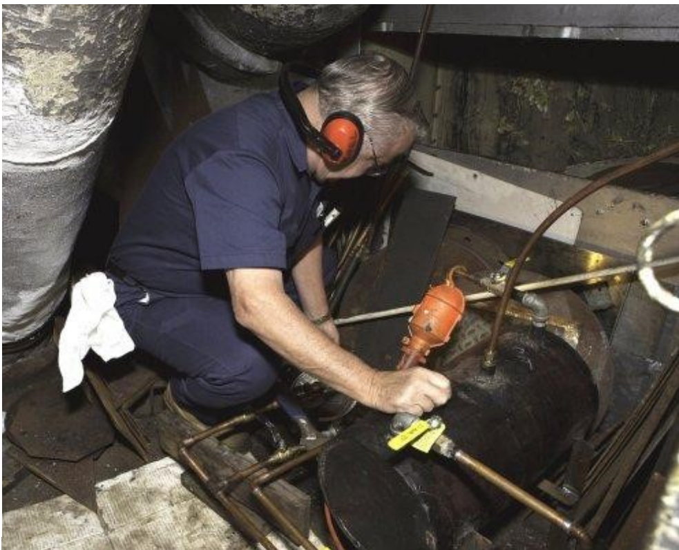
Karl Herchenroder works on heating system repairs.
