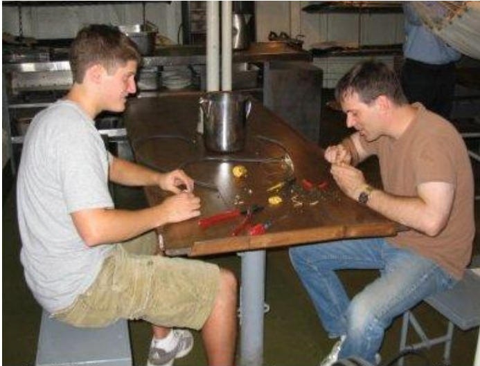
Electricians Ben Waxman and Barry Witte on the messdeck refurbishing electrical parts.
