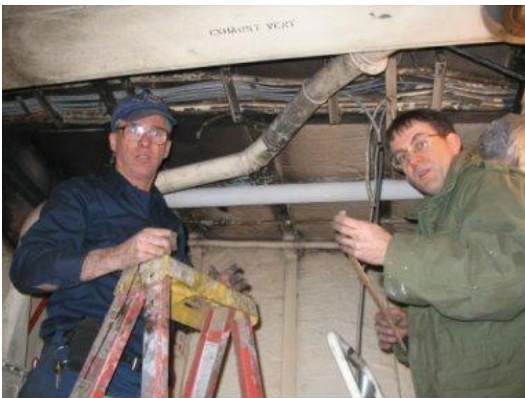
Gary Sheedy and Barry Witte replace burned cables.
