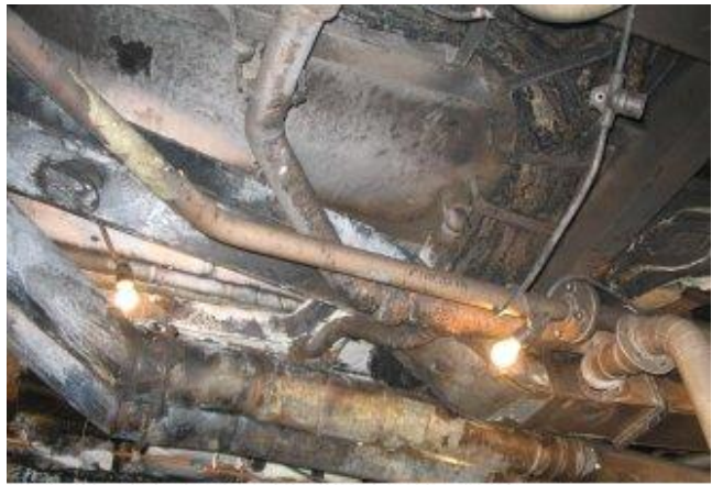
Overhead fire damage - starboard side.
