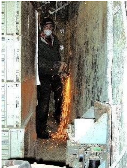
Gary Sheedy doing the final scaling in the electrical storeroom.
