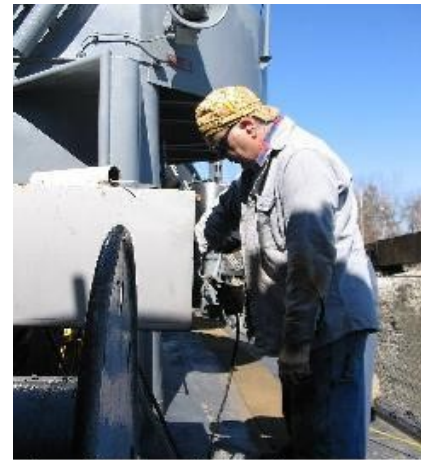
Doug Tanner welding up the new stainless steel septic tank.
