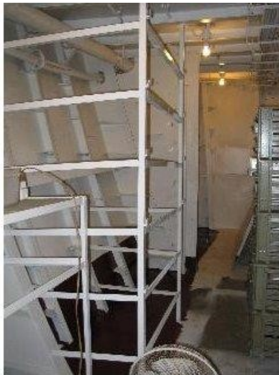
The storeroom after the bulkheads were sprayed.
