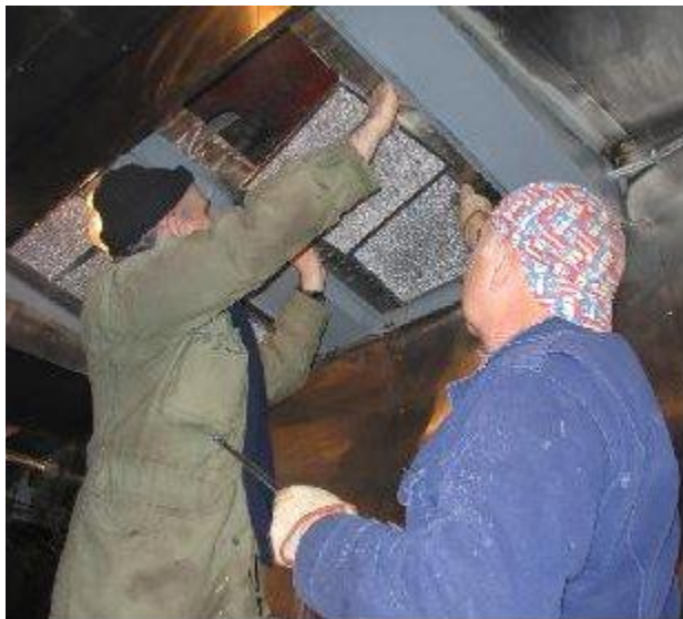
Chuck Teal and Doug Tanner installing grease screens above the new galley stoves.
