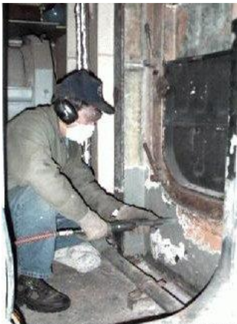
Jim Gelston hard at work chipping the laundry.
