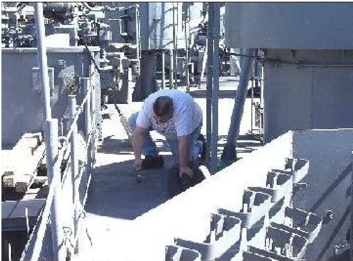
Scraping the 01 level.
