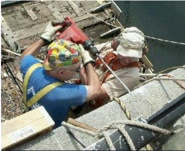
Doug and Tim drilling for the gangway.
