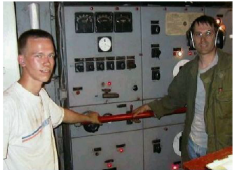
Electricians Mike Clark and Barry Witte.
