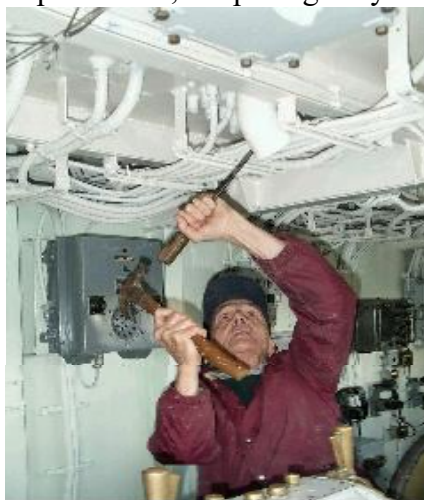
Larry Rocky Rockwood putting the finishing touches on the pilothouse.
