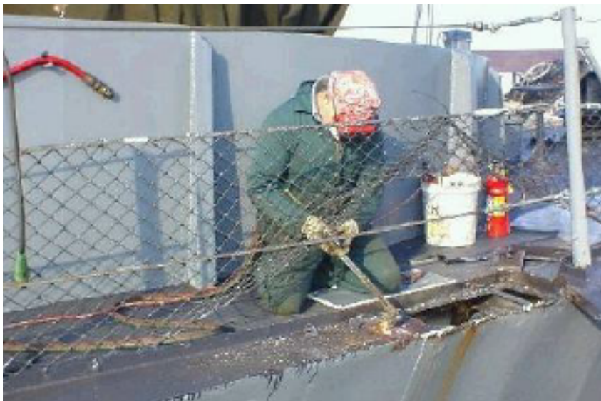
Tanner cutting out wasted metal under a chock.
