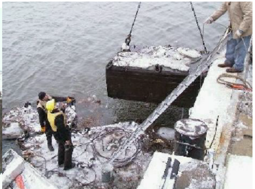
Making another lift.
