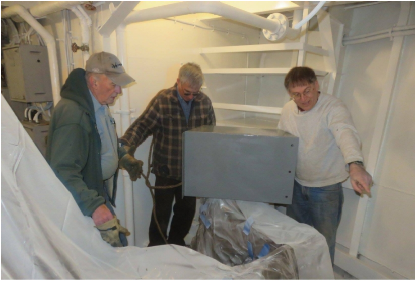
Barry Witte getting ready to install the smoke generator tank that his students fabricated.
