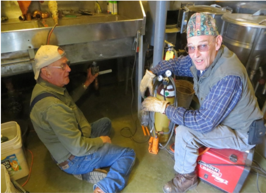
Andy Sheffer and Tim Benner working on the galley sink drains.
