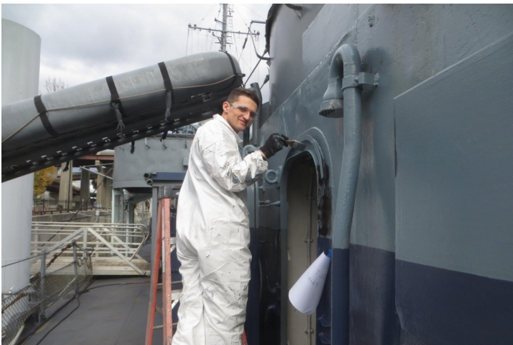
Touching up some new metal following Ed Zajkowski's work week.
