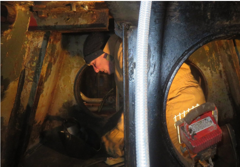
Danny Statile finishing the welding under gun three.
