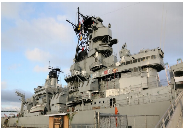
USS IOWA in San Pedro. I'm glad I didn't have to paint her.
