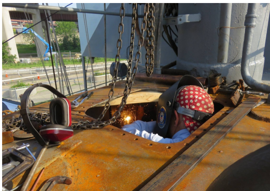
Progress on the RDF platform.
