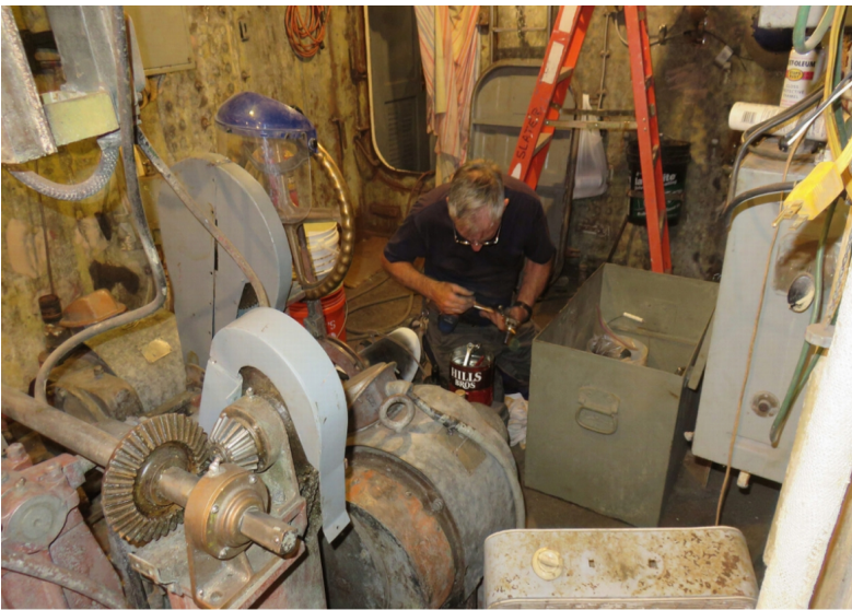
Gary Sheedy making progress in the steering gear room.
