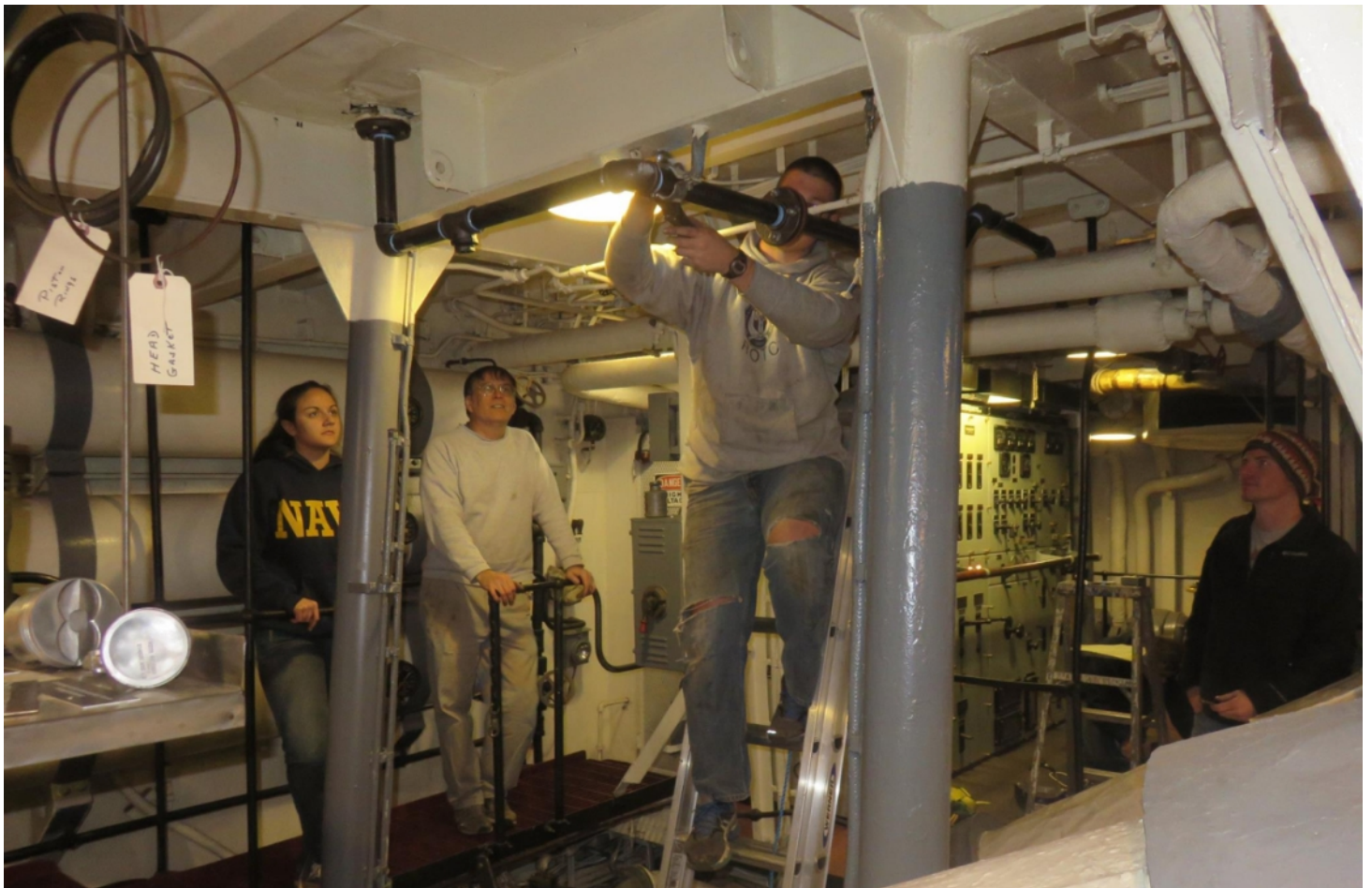
Midshipmen working on the firemain.
