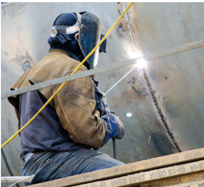
Seal welding the waterline doubler.
