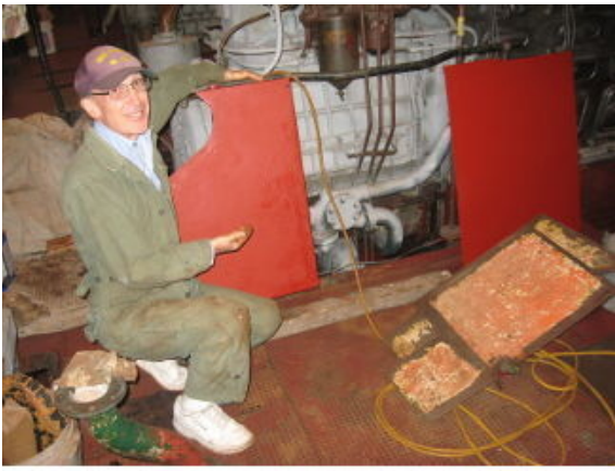
Gary Dieckman painting the underside of the deck plates.
