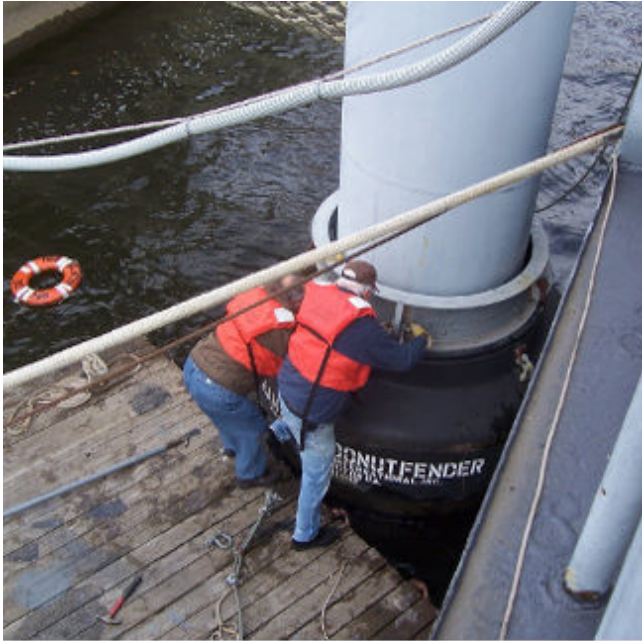
Walt Stuart and Chief Smith connecting the spring wires to the dolphin collars.
