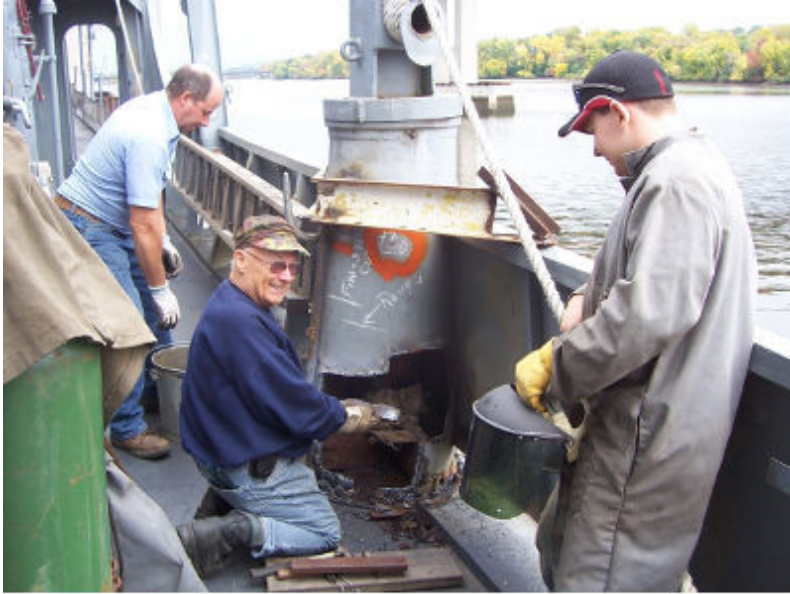
Progress on the davit pedestal project.
