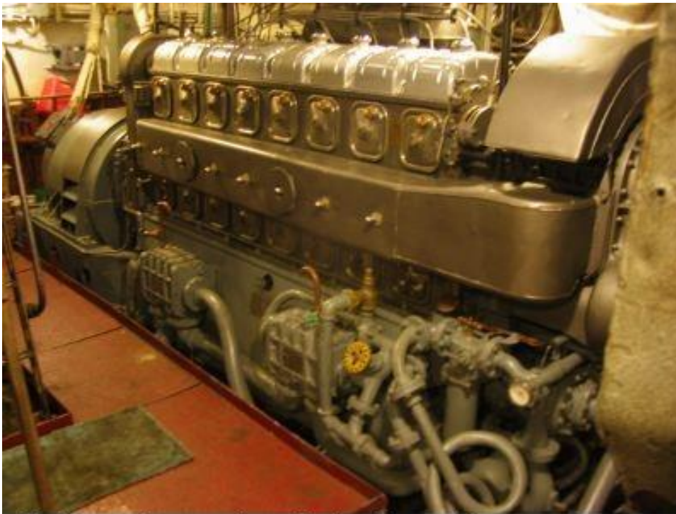
All cleaned up and ready for the public.
