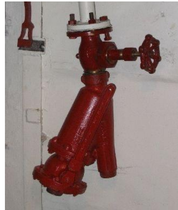
"Super" Dave got the messdecks strainer right, if he just remembers to tighten the bolts.
