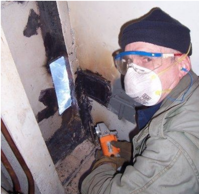
Chuck Teal looking through our new hole at the ice in the river below as he fits a new patch.
