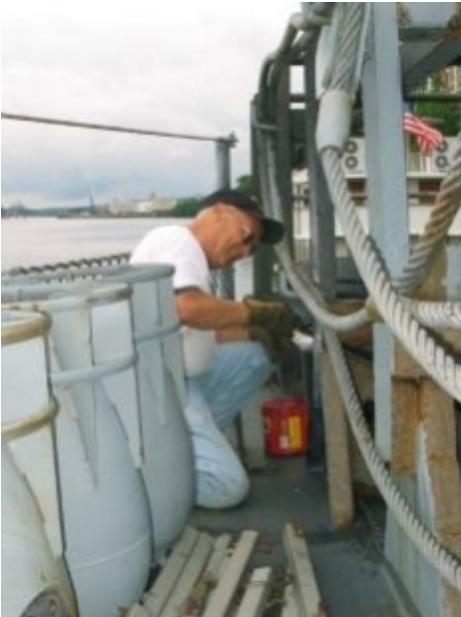
After chipping Dave applies Coraseal to help prevent the rack from rusting!
