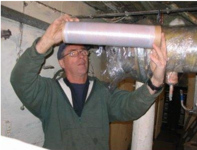
Garry Sheedy masks the copper tubing and other fittings on the reefer deck in preparation for painting.
