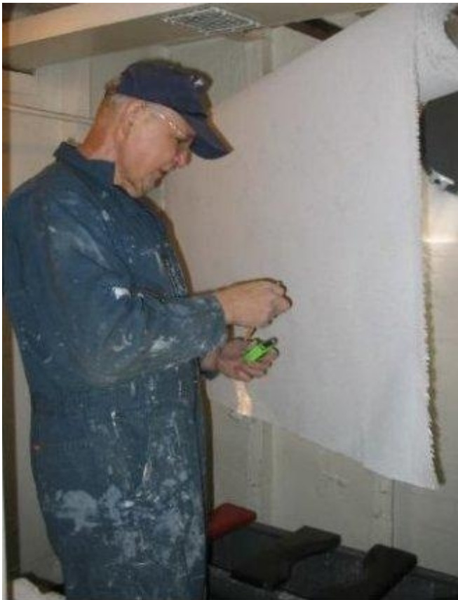
Stan Murawski measures cloth insulation covering for the log room.
