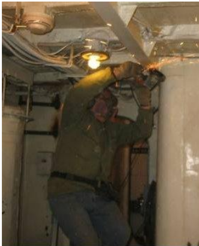
Gene Jackey grinds off excess metal in the washroom.
