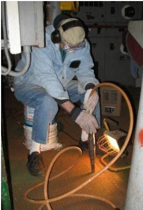
Don Miller works to chip years of gunk off the aft motor room deck.
