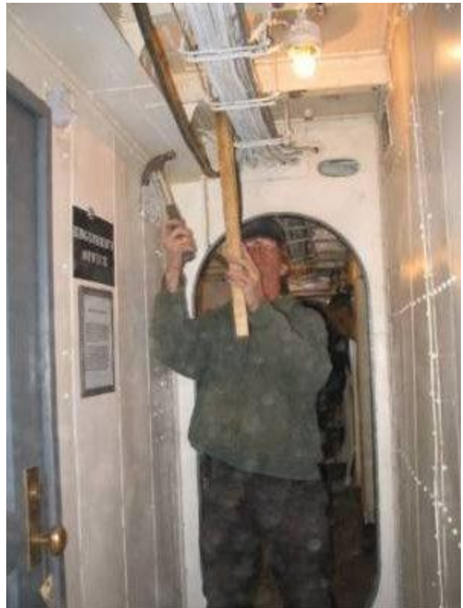
Gary Sheedy knocks overhead cables back into position - neatness counts!
